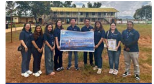
Behn Meyer Myanmar Supports the Renovation of Earthquake-Damaged Schools in Shan State
